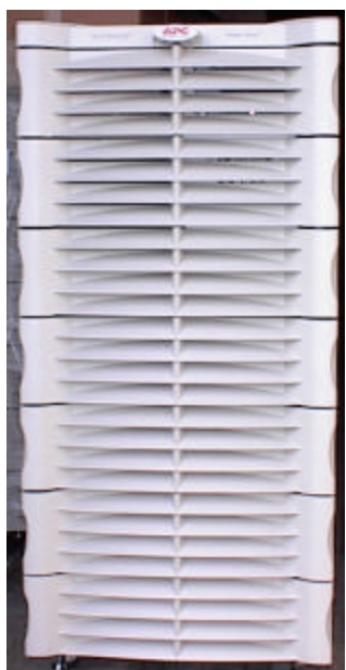
Figure 7: APC Operations Room UPS System
