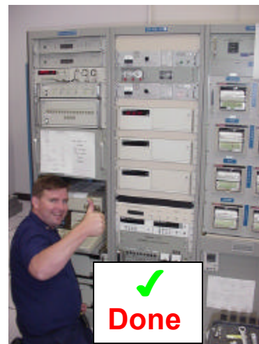
Figure 3: New Cesium Beam Oscillators and TTM Equipment (LORSTA Havre, MT)
