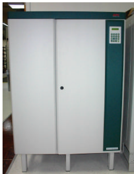
Figure 8: APC Transmitter UPS System
